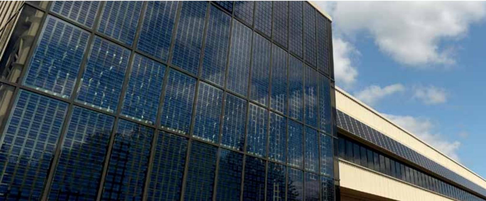
Building Integrated PV uses solar photovoltaic panels to replace conventional building materials in the roofs, walls and sun shading of buildings. The practice of integrating Solar PV modules to enable buildings to generate electricity is increasing in popularity as the technology improves and costs reduce.
