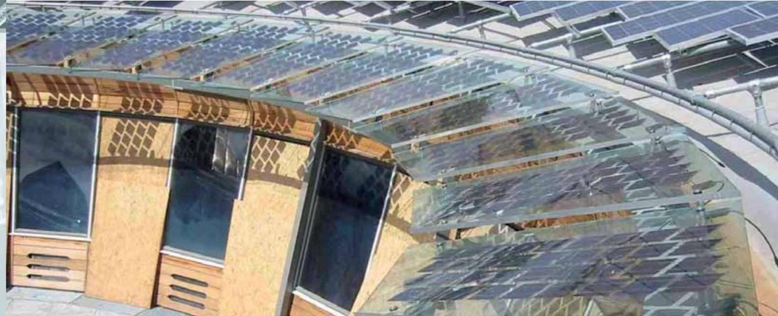
PowerGlaz® BIPV is mainly used on glazing elements within the façade or roof structure but this is by no means the only application.
