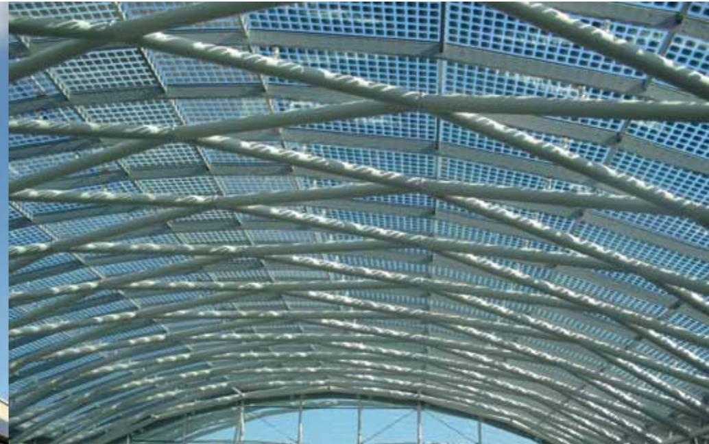
Our extensive experience in glass processing means that we process all the glass components used in PowerGlaz® BIPV and this enables us to offer single glazed panels or double-glazed units which comply with building regulations.
